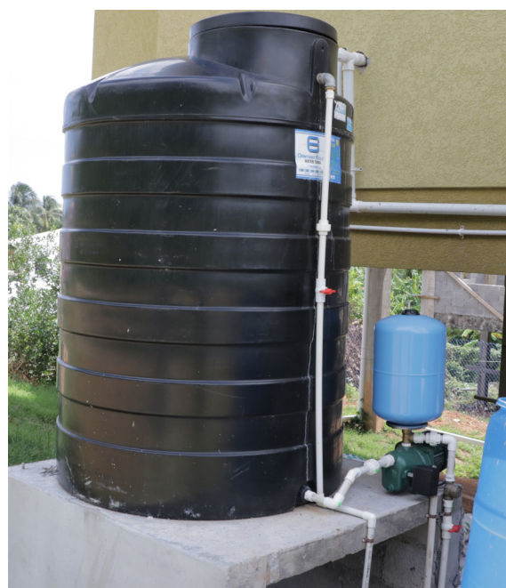
EDA Water Storage Tank Project
